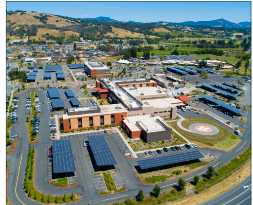
Ameresco's partnership with Sutter Health Santa Rosa advances sustainability initiatives with solar power to optimize energy usage and improve patient care. The 1.6 MW of solar offsets 40% of the hospital's overall electricity usage.
